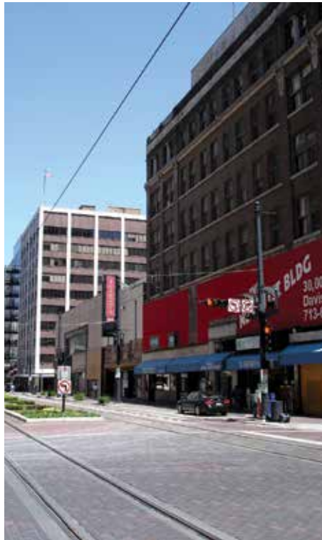
The original site was one of the most blighted blocks in downtown Houston.
