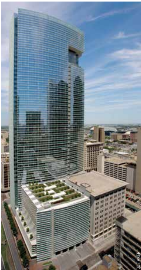
Sited on three-quarters of a block, BG Group Place shares the block with an existing building with historic qualities (on the right) that is being planned for reuse as a hotel by another developer.
