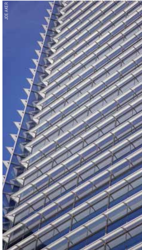
The facade includes horizontal sunshades—two shades per floor—of glass and aluminum that wrap around the north and south facades. The building has been certified LEED Platinum by the U.S. Green Building Council.
