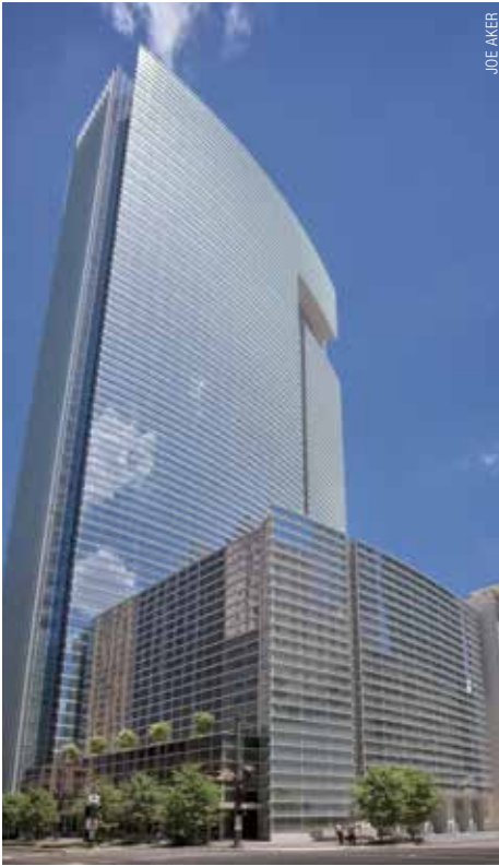
The parking garage is completely enclosed behind a glass curtain wall.
