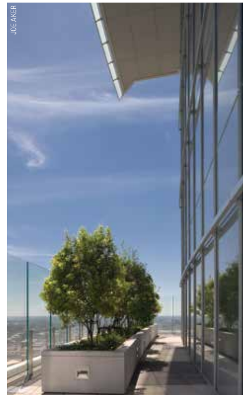
The sky garden, which spans floors 39 to 43.
