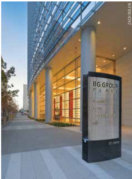
The atrium glass along the front, together with landscaping, creates an attractive pedestrian experience along Rusk Street.
