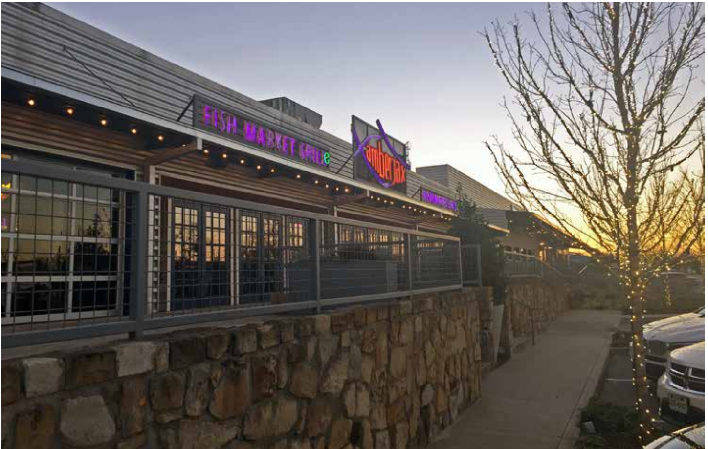
On its north side, the Old Terminal Building features both the Amberjax restaurant and the new Hall restaurant, as well as the Cake Bar and Kate Weiser Chocolate.
